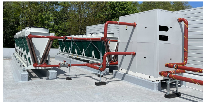
Dedicated chillers for Hortense, on roof of UGent datacenter S10, a.k.a. "loopC"
